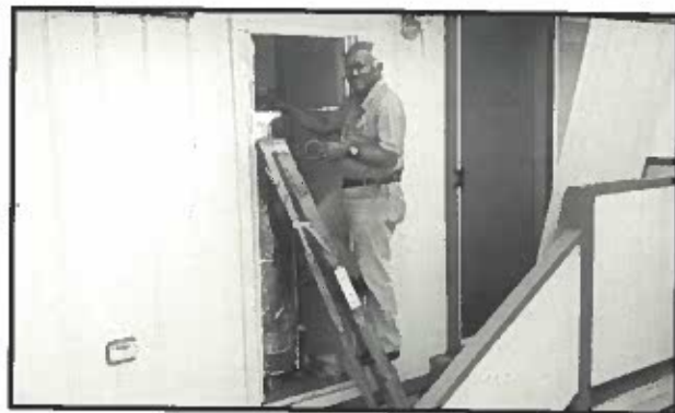
Fred Baisa on-the-job, securing a water heater blanket for a client.
