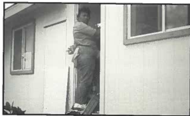
Doreen Galam, MEO Molokai's energy person, installs a heater blanket.
